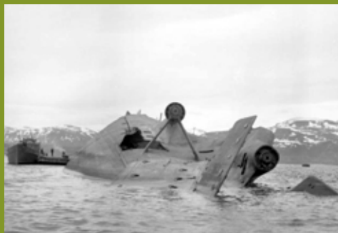
The German battleship Tirpitz, lying capsized in Tromsø Fjord, attended by a salvage vessel. The hole in the hull by the starboard propeller shaft was cut by the Germans to allow access to salvage crews.
