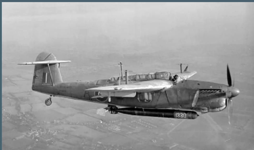
A Royal Navy Fairey Barracuda II (s/n P9926) from Lee-on-Solent Fleet Air Arm Station, Hampshire (UK), with torpedo, in flight. The wooden plane that steadied the torpedo before it struck the water and broke off can be clearly seen at the rear of the weapon. Photo: Wikimedia Commons (Public Domain).
