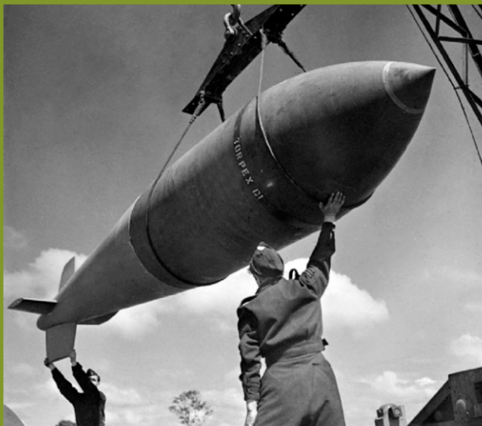
A 12,000 lb Tallboy bomb is hoisted from the bomb dump to its carrier at Woodhall Spa, Lincolnshire, to be loaded into an Avro Lancaster. Photo: Crown Copyright (Public Domain).
